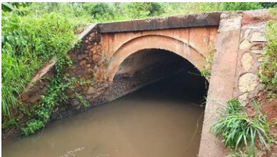
Photos 53: Pont Arche
